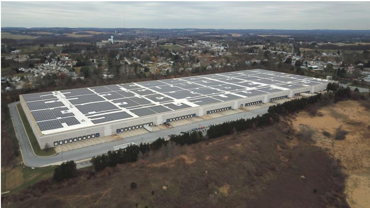
Covering the 23-acre roof of a building owned by STAG Industrial, Summit Ridge Energy's rooftop community solar project in Hampstead is capable of generating 9.2 megawatts, providing monthly energy savings to approximately 1,300 residential and small commercial customers located across the state. (Dylan Slagle)
