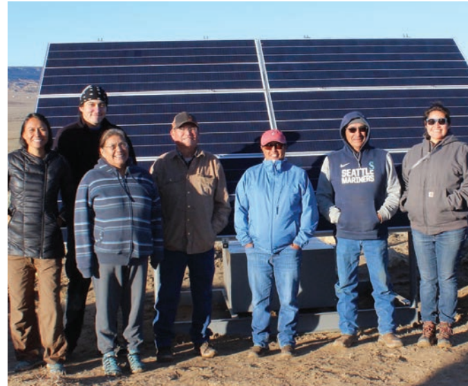
Off-grid solar PV system installation by Native Renewables team (courtesy of Native Renewables).
